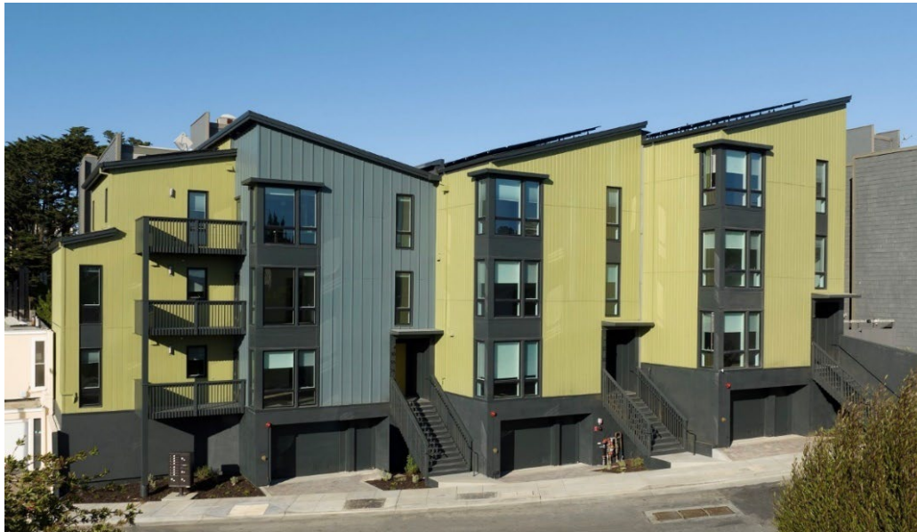
Habitat for Humanity Greater San Francisco homes in Diamond Heights, San Francisco
