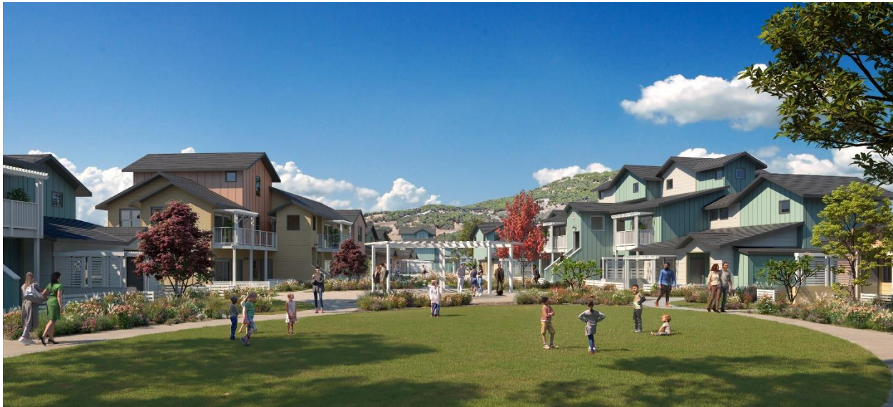
Habitat Greater San Francisco's newest affordable home development along Redwood Blvd in Novato, Calif.
